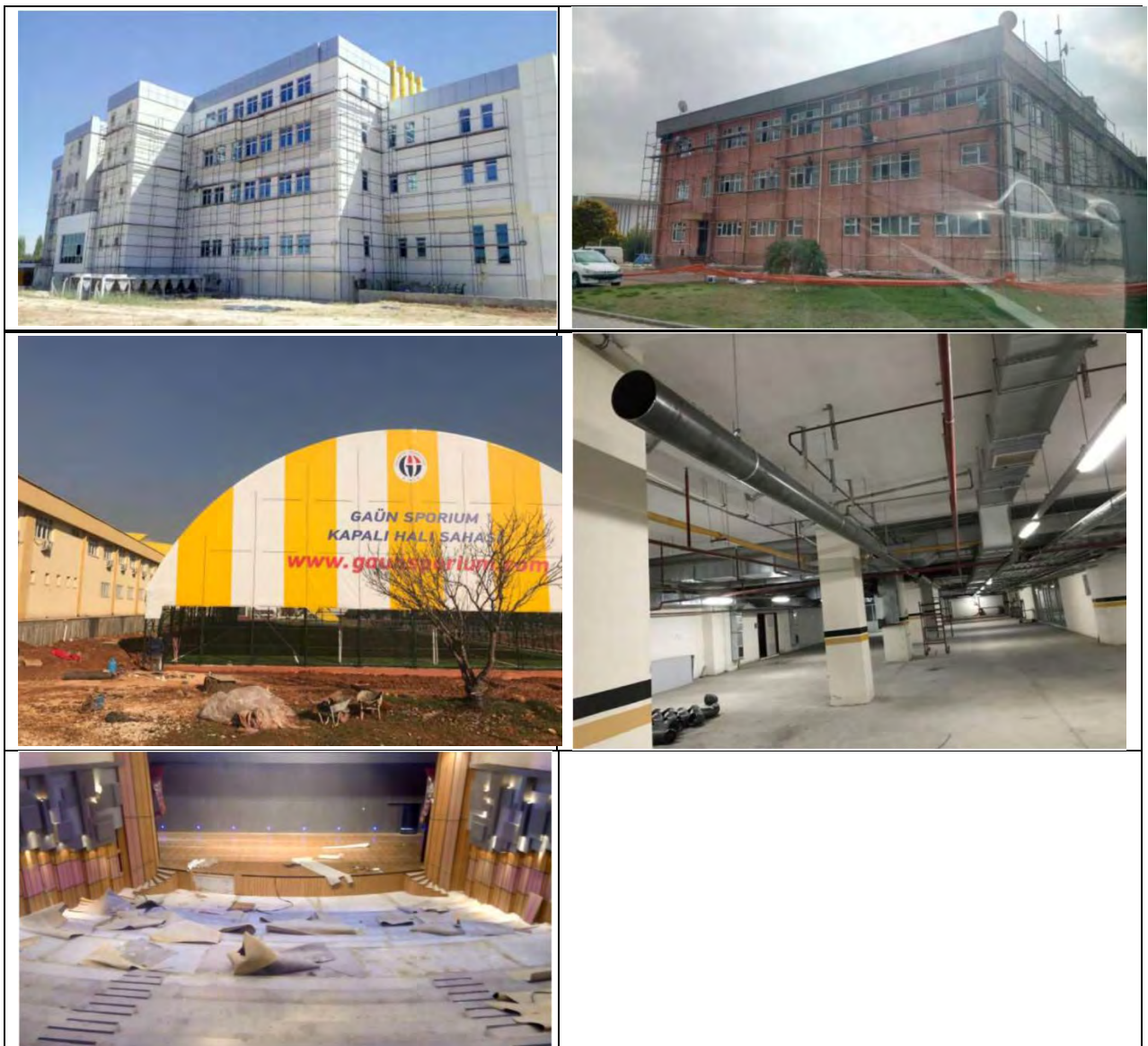
Example of operation and maintenance activities during Covid-19 pandemic in Gaziantep University (Engineering Faculty, Sport centre, Congress Centre, Faculty of Dentistry Water reservoir and Pipes)
